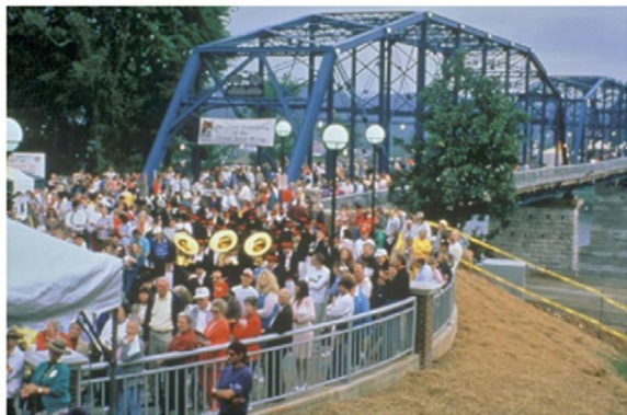
Reopening of Walnut St. Bridge in 1993 Photo Courtesy of the RiverCity Company
